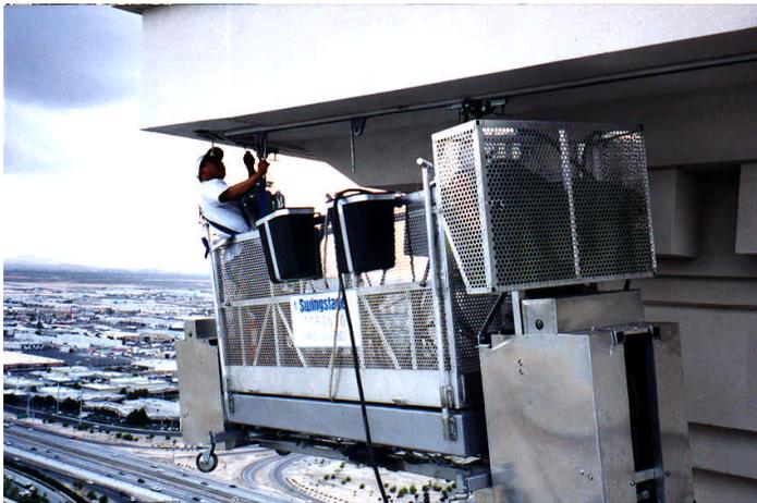
Example of Monorail used to suspend a TRACMOD Powered Platform
